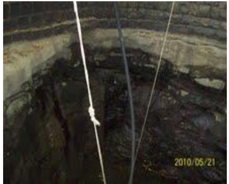
Photo 5.2 Dug well with compact Zeolitic basalt with subsurface springs
